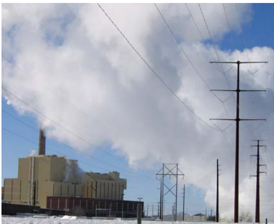
The GCMW Transmission Line at the Weston Power Plant
