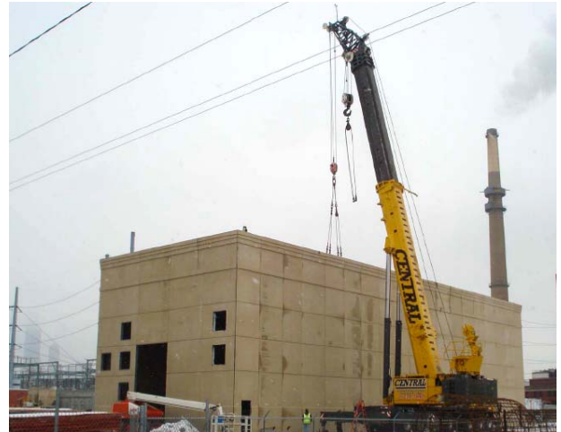
345 kV GIS Building under Construction
