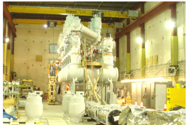
Installation of 345 kV GIS Equipment
