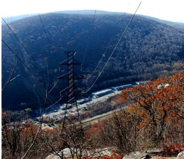
Existing River Crossing Span
