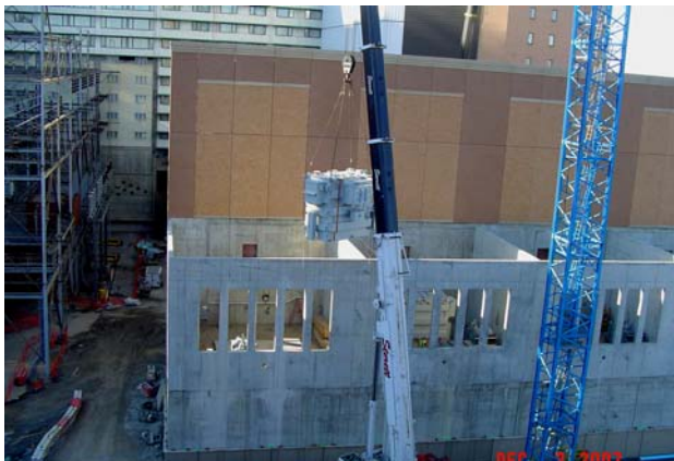
138-13.8kV Transformer Being Placed in the Waterside West Substation Enclosure
