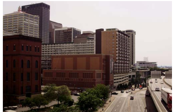
Waterside West Substation Viewed from Second Street Bridge
