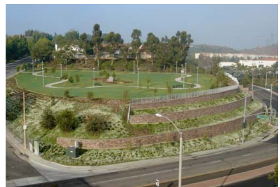
Roosevelt Park Conceals the Completed Park Substation
