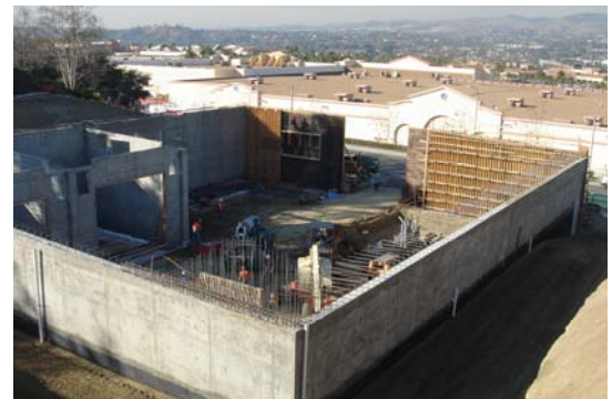
Construction of Park Substation Enclosure
