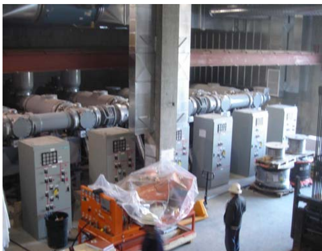
Interior of Park Substation During Construction
