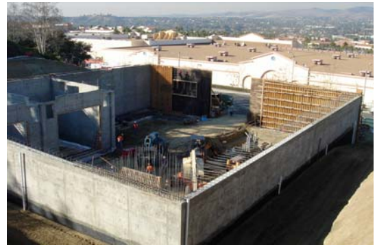
Construction of Park Substation Enclosure
