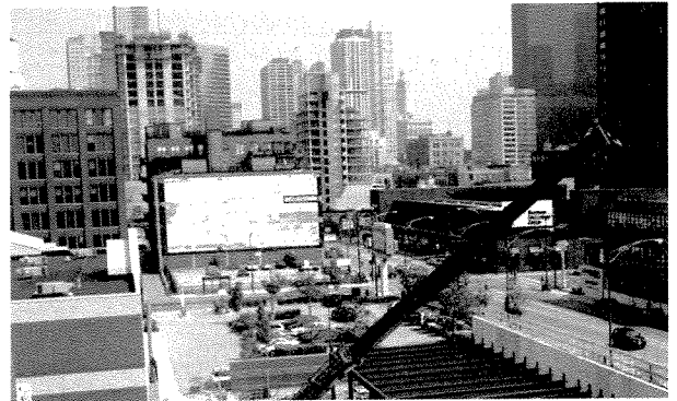
ComEd's "Chicago Optimization Plan to the City" include the construction of the Madison Substation which is underway in downtown Chicago.
