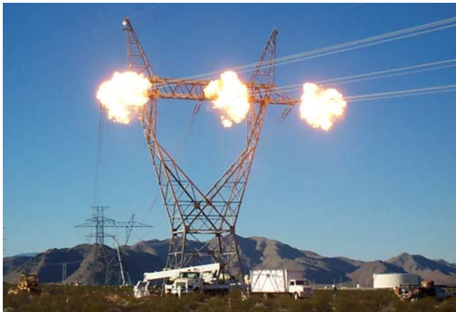
Installation of Implosive Deadend Fittings
