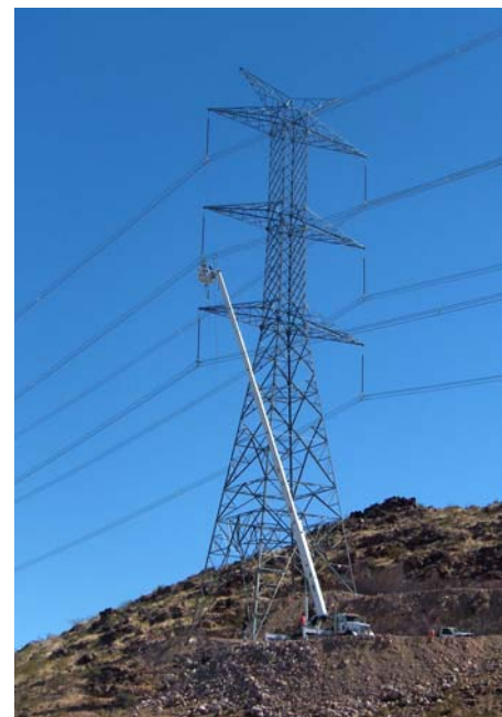
Clipping-in Conductors on Double-circuit Towers
