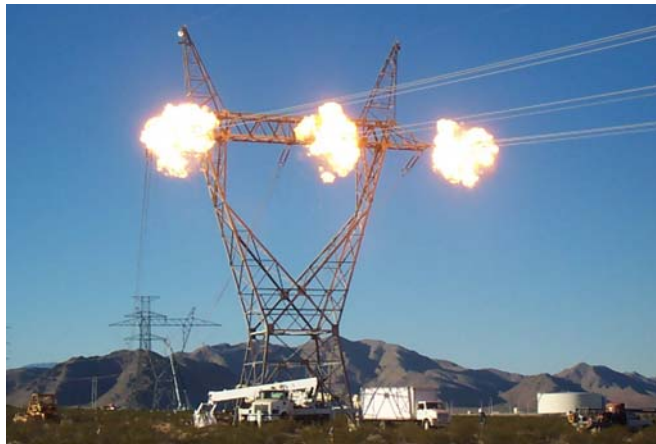
Installation of Implosive Deadend Fittings
