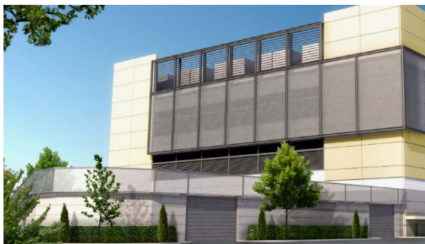
Rendering of Collman Substation Enclosed by a Decorative Wall (Echelon Place Main Plant in Rear)
